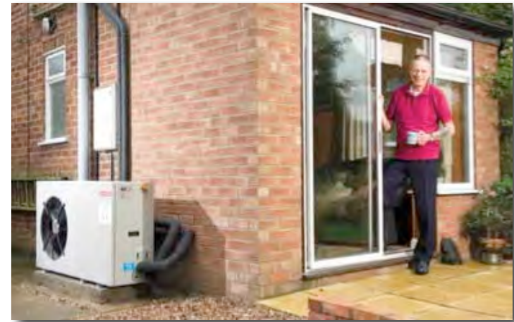
Air-source heat pump
