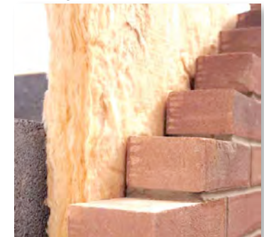
Cavity wall insulation
