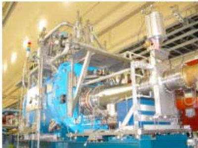
The superconducting cavities will be upgraded to absorb more higher-order mode power up to 50 kW.
